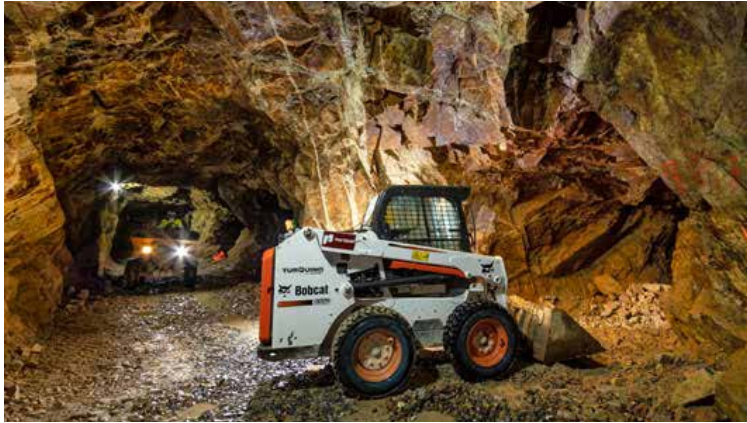
Rafaella completed a recommissioning study for the underground complex at its Santa Comba tungsten-tin project in July
