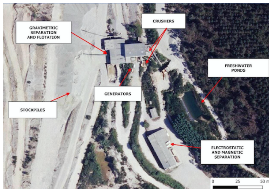
Figure 43: Aerial view of the main facilities at San Finx
